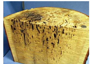
Picture 3: Carpenter ant damage to wood.
